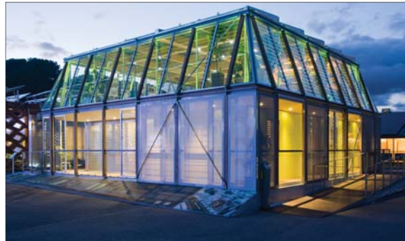
The winning Canopea House from Team Rhône-Alpes was a prototype of the top two levels of a tower: one home and the common space above.
