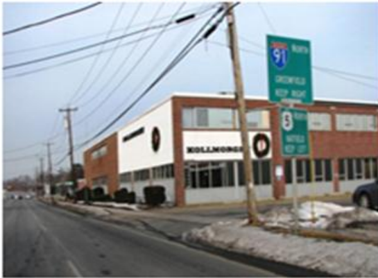
MAIN BUILDING NORTHAMPTON, MA
