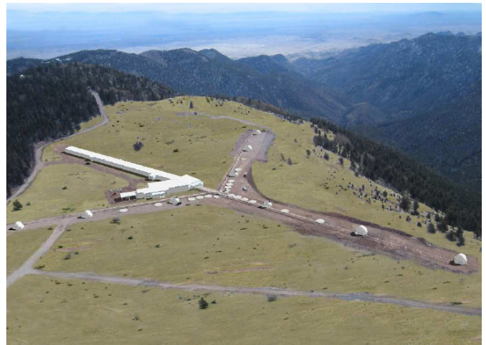
Figure 1. Architectural rendering of the now-completed Magdalena Ridge Observatory Interferometer (MROI) delay-line facility and beam-combining laboratory (as well as the as-yet-unfinished telescopes) atop Magdalena Ridge. The telescopes will be movable onto 28 pads, with separations ranging from 7.5 to 340m.
